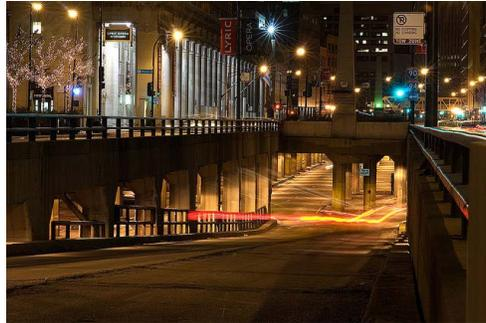
Wacker Drive is a double-deck configuration, featuring a city street above and uninterrupted traffic flow beneath.
